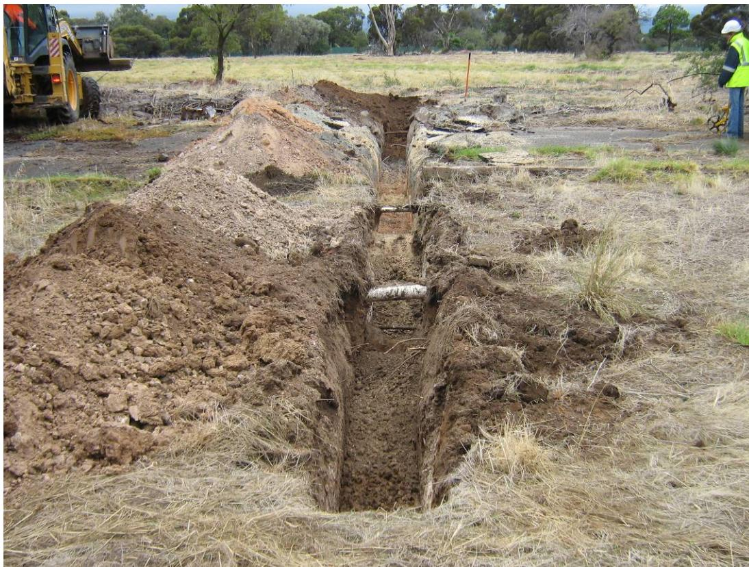
**Photo 7      Trench 2 showing the numerous underground services intersected**
