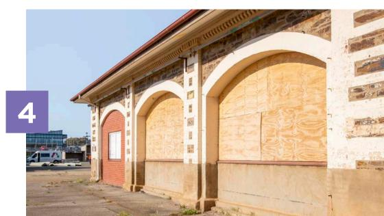
This random rubble and red brick structure, built in 1873, was originally used for gas purification. After the Second World War the interior was adapted to serve as storerooms, laboratories and amenities rooms for workers.
